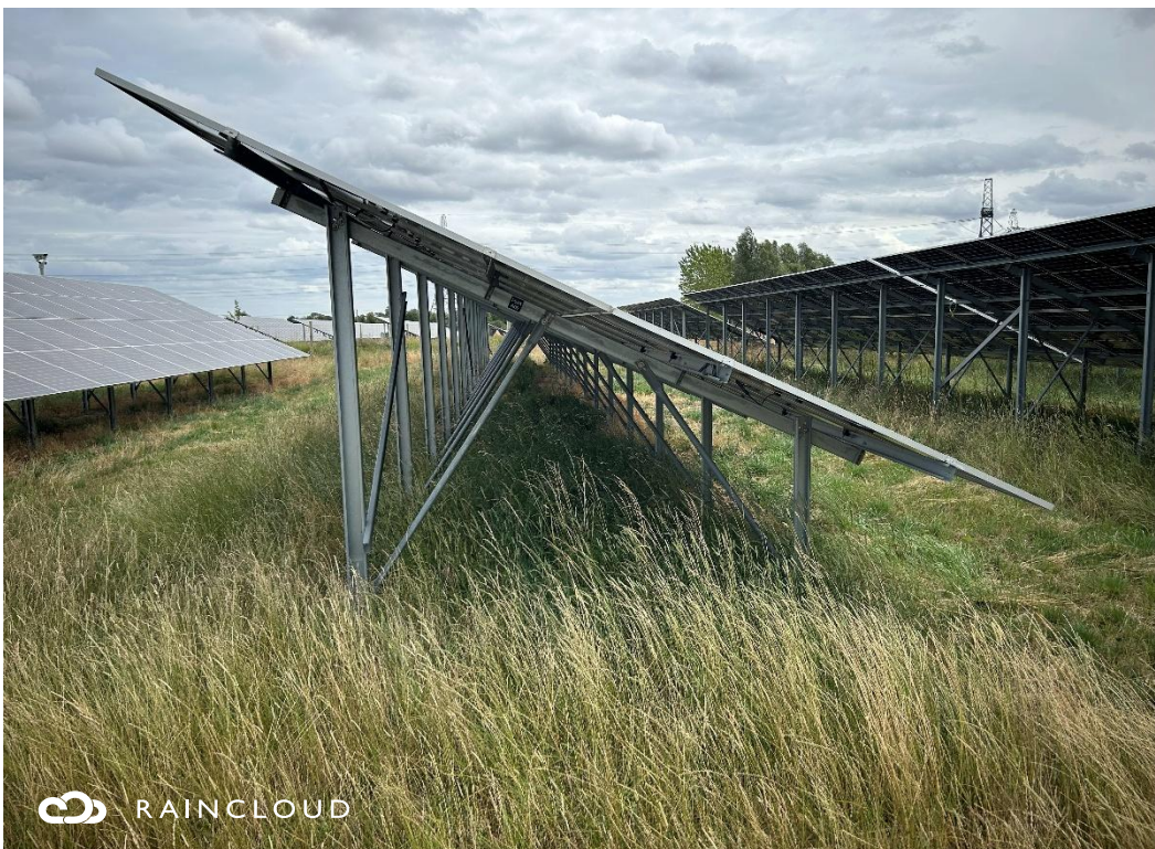
Plate 12-18 Thin PV Racking Mount
