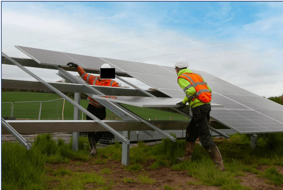
Plate 12-24 PV module installation (Ref. 12-16)
