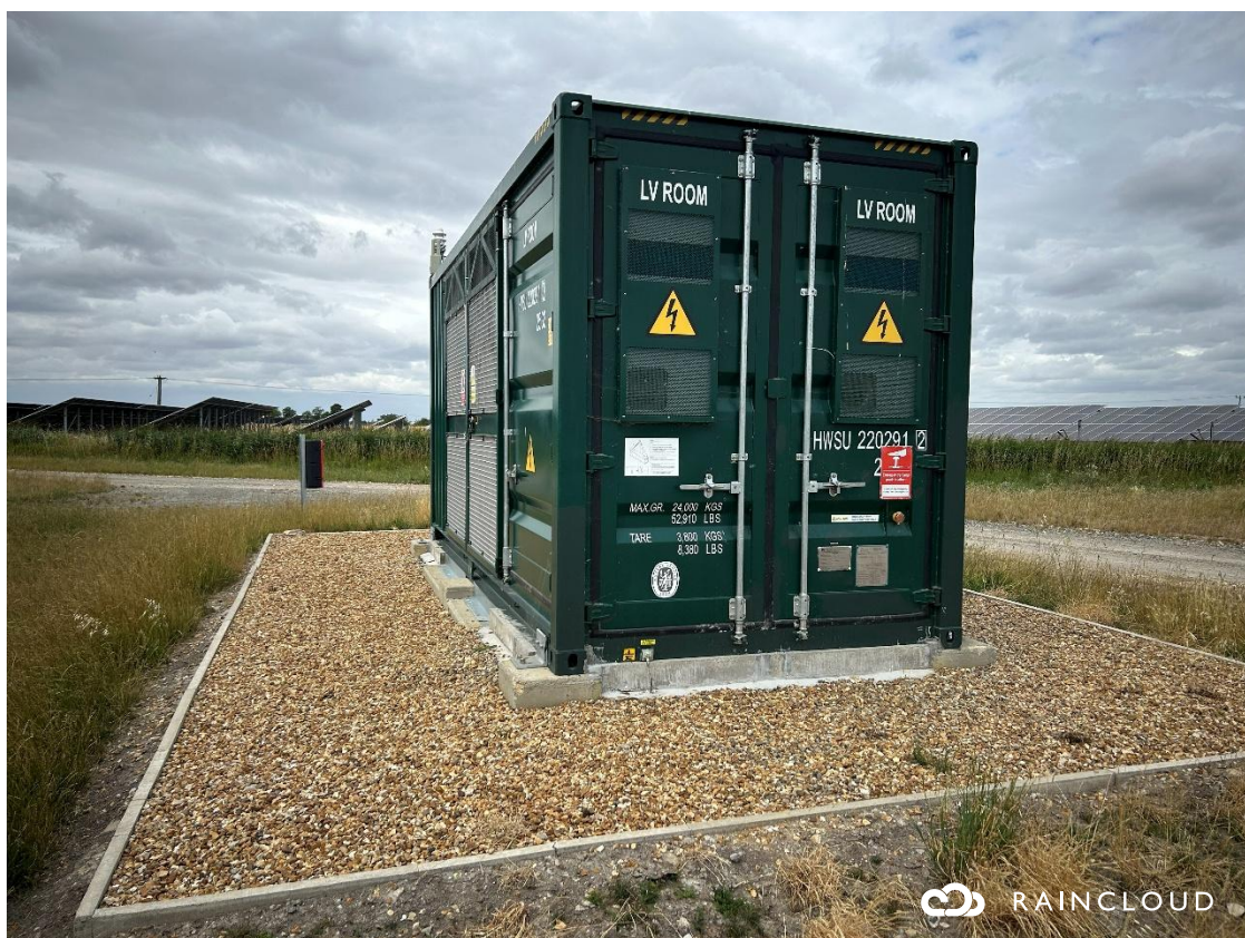
Plate 12-33 Conversion unit gravel surround
